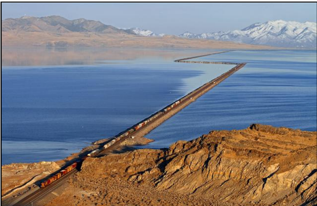
Going to sea by rail: An eastbound Union Pacific freight begins the long trek across Great Salt Lake at Lakeside, Utah, as the end of the train in the foreground is about to leave terra firma for the long 20-mile trip across the causeway. A wood trestle used to carry the line straight across in front of the train, but was later replaced with the fill that now zig-zags 1,500 feet to the north. Promontory Peninsula and the Wasatch Mountains dominate the background, with Ogden located between them.
