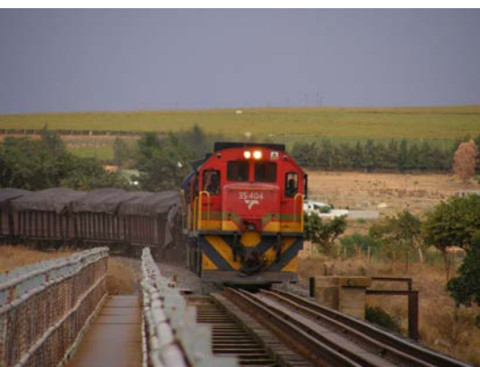
Crossing the Berg River Bridge at Moravia.
