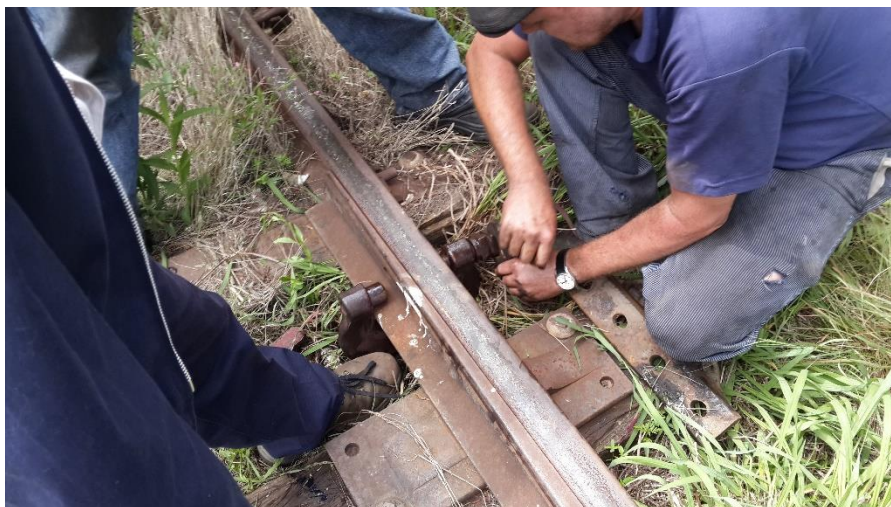
Track repairs at Magaliesburg.
